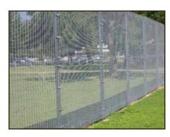
Heavy gauge welded wire fence mesh is the preferred solution for perimeter protection of sensitive sites. The small mesh openings discourage climbing by eliminating toe and/or finger holds. Additionally, welded wire mesh will not unravel or lose structural integrity when cut. Creating an opening in the mesh is time-consuming and difficult. The corrosion-resistant mesh can also be buried to discourage access from below.
